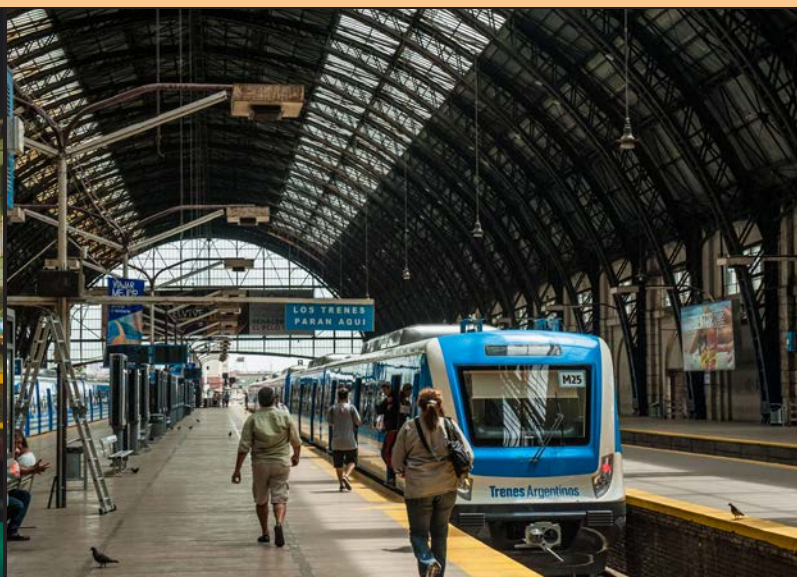
Argentina's Retiro Linea C station in Buenos Aires, sports a classic dome structural design with metal webbing, typically found in many European cities. This line runs north to Tigre, gateway to the rivers and wetlands of the vast Paraná River delta. The recently replaced train sets, are made in China.
